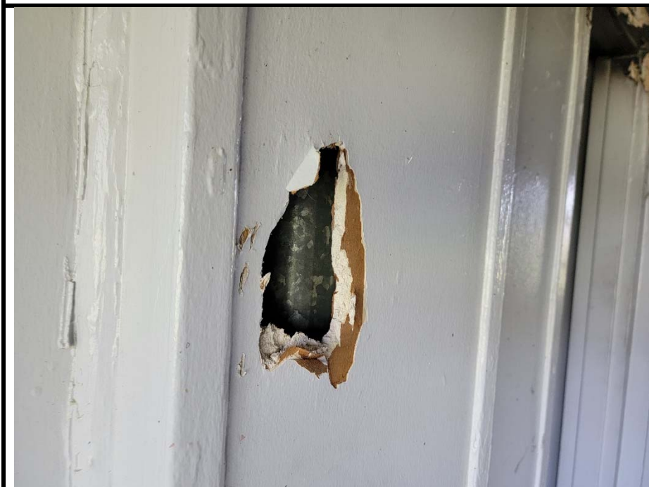
6. Non-ACM Drywall at Duct Chase
