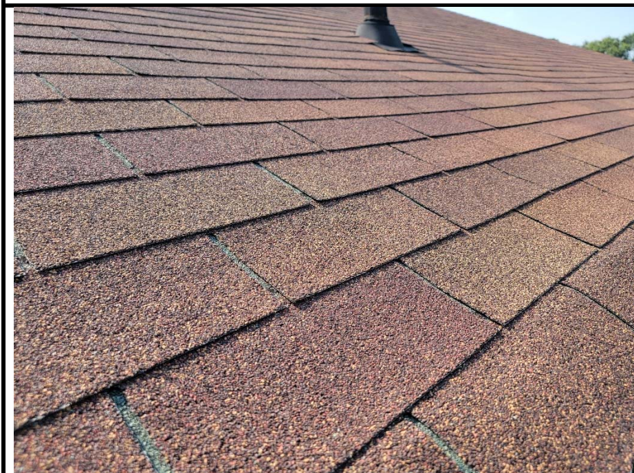
12. Non-ACM Asphalt Shingle Type 1
