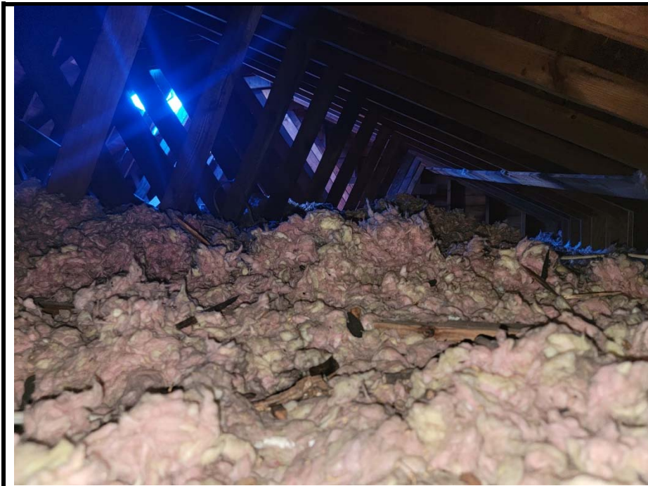
5. Fiberglass Fill Attic Insulation
