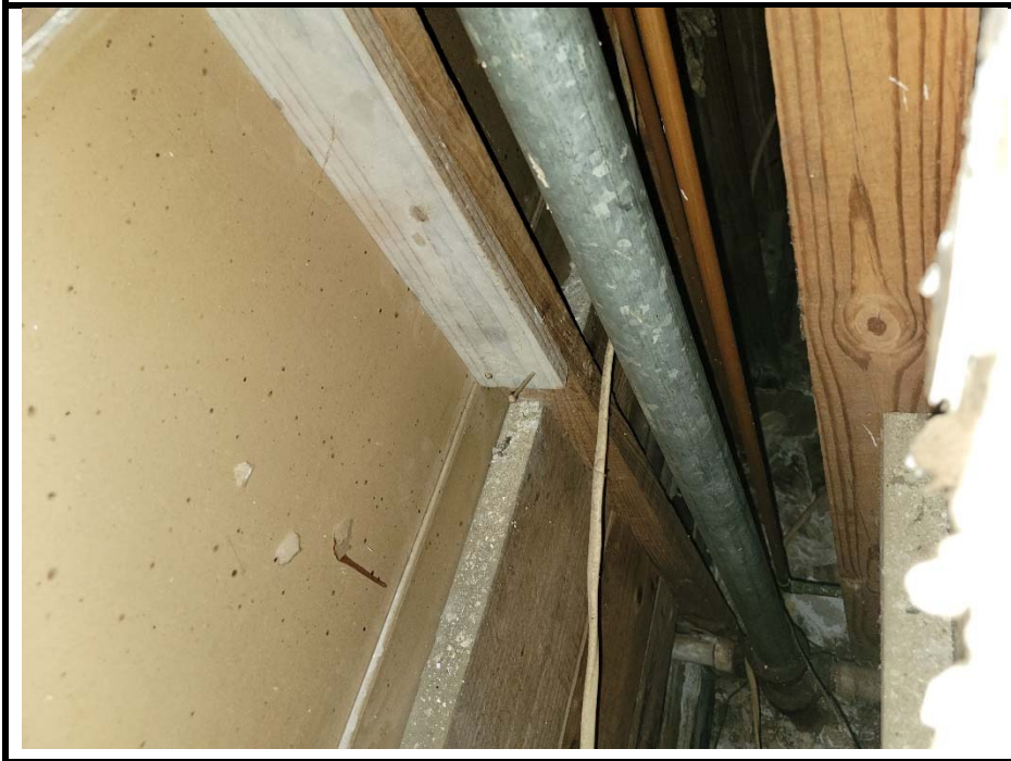
8. Non-ACM Plaster Board Bathroom Walls
