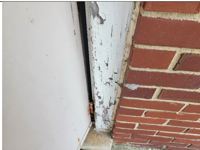
Original LBP Wood Door Casing/Jamb (often below Aluminum)
