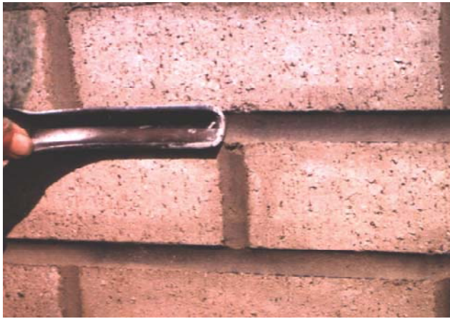
Photo 4 Concave Mortar Joints
