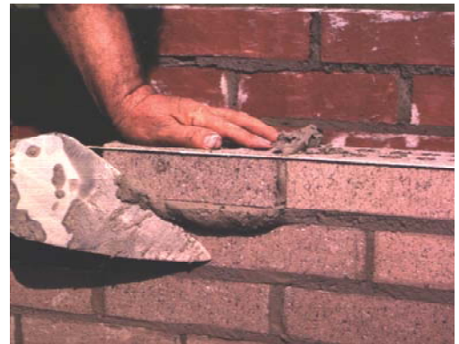
Photo 2 Cutting Excess Mortar
