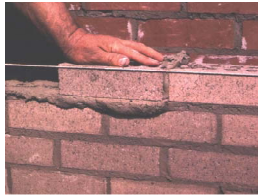
Photo 1 Shoving Brick into Place
