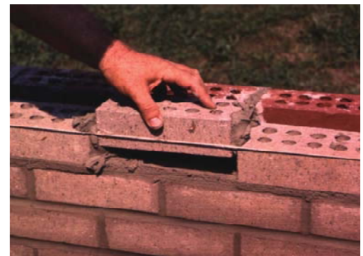
Photo 3 Placing the Closure
