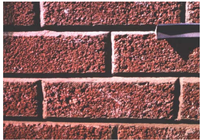
Photo 5 "V" Mortar Joints
