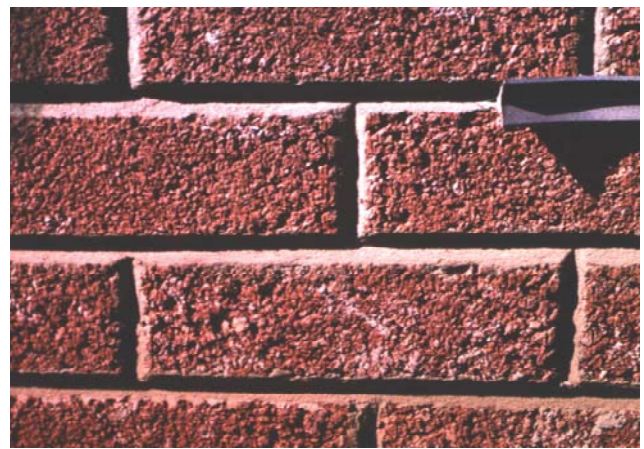
Photo 5 "V" Mortar Joints
