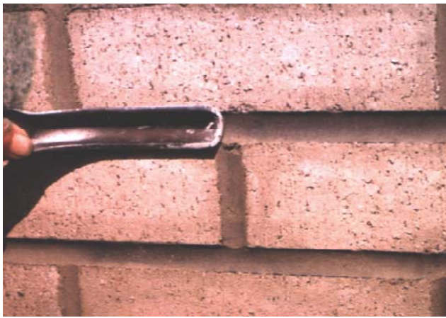
Photo 4 Concave Mortar Joints
