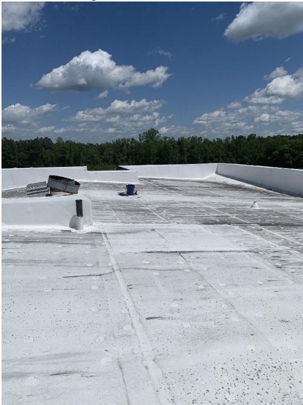
Roof, Building A TPO Membrane
