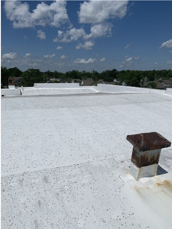
Roof, Building A TPO Membrane
