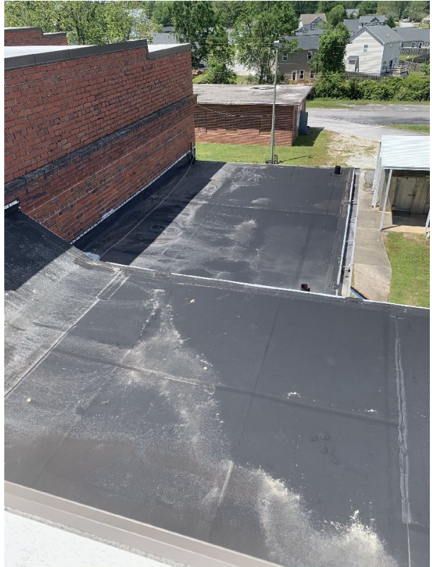
Roof, Building A EPDM Membrane
