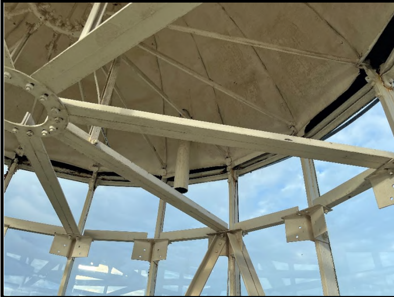
9 White structural steel located on the 9 th landing level tested positive for lead-based paint (8% wt).
