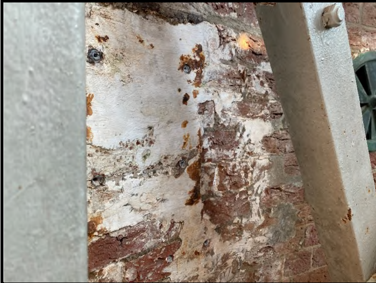
5 The block filler coating tested negative for asbestos and PCBs.
