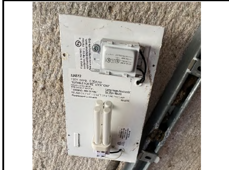
12 View of small fluorescent bulb located on the first landing level with an electronic ballast.
