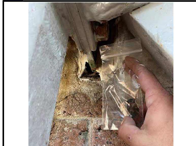
4 The white caulk located between the structural steel and brick on the 8 th landing level tested negative for asbestos.
