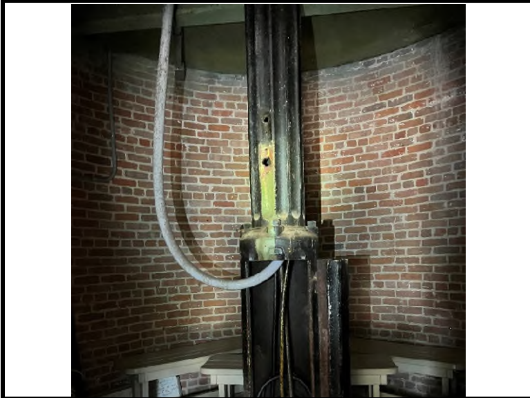
7 The metal central stairway support/conduit located on all levels tested positive for lead-based paint (1.2% wt).
