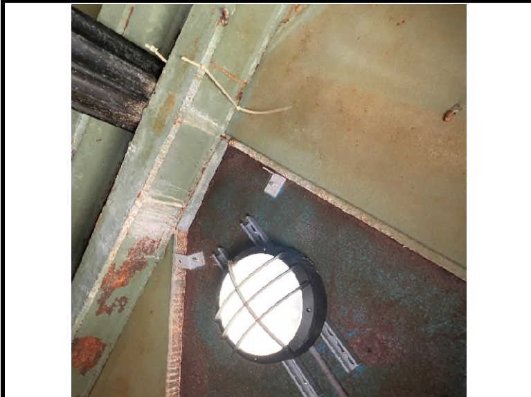
11 View of light fixture containing a CFL bulb.
