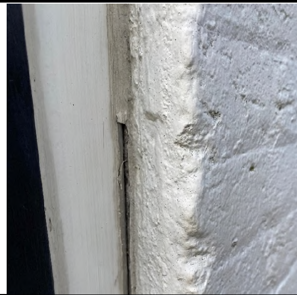
6 Various caulks associated with the structure tested negative for asbestos and PCBs.
