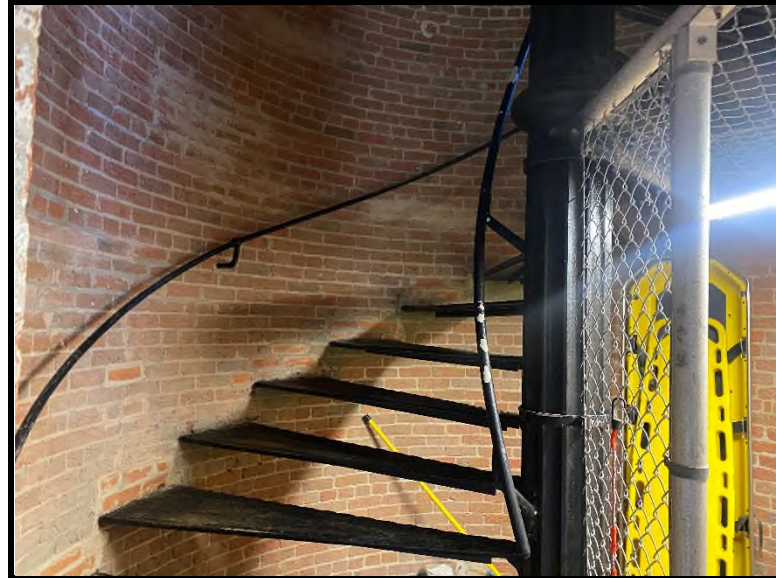
10 The black metal handrails and interior stairs tested positive for lead-based paint (0.91% wt).
