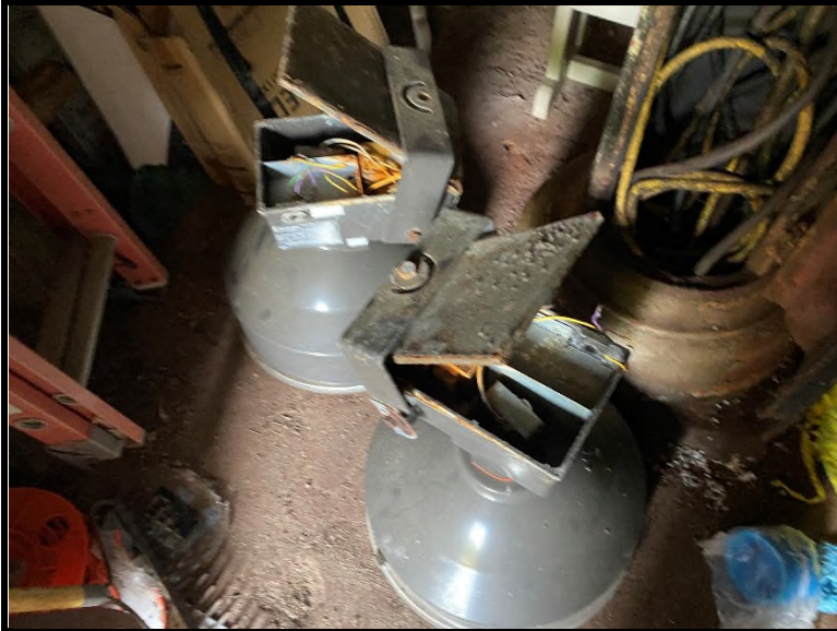
13 View of two light fixtures with potential mercury vapor bulbs. The ballasts associated with the fixtures are presumed to contain PCBs.
