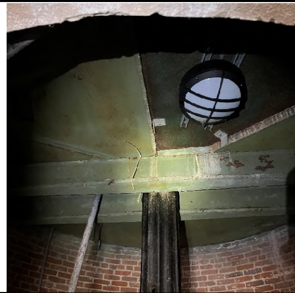
8 The metal ceiling and structural steel on the first landing level tested positive for lead-based paint (10% wt).
