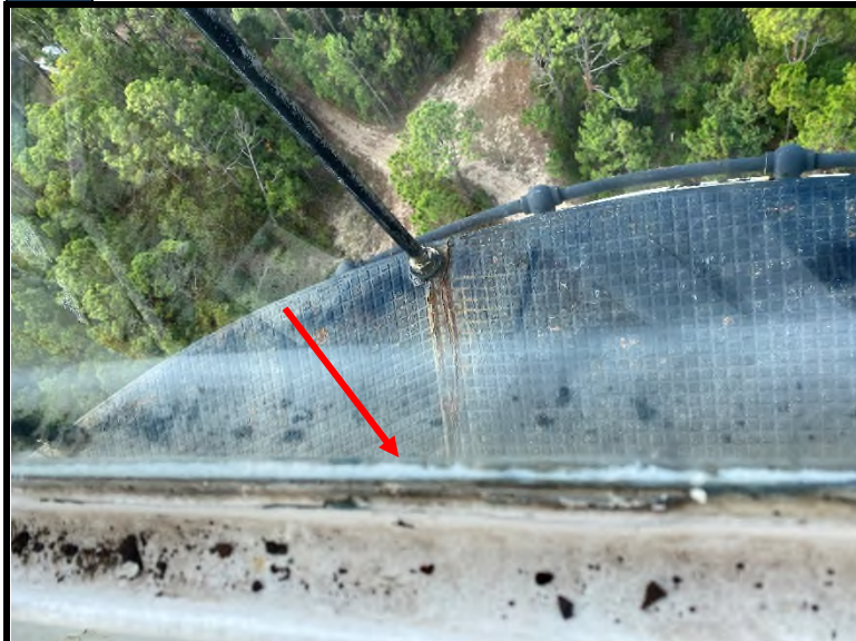
3 View of the inaccessible window glazing located on the exterior of the windows on the 9 th landing level. The window glazing is presumed to contain asbestos.
