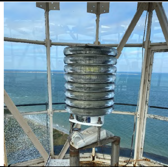
14 View of the LED light associated with the lighthouse.
