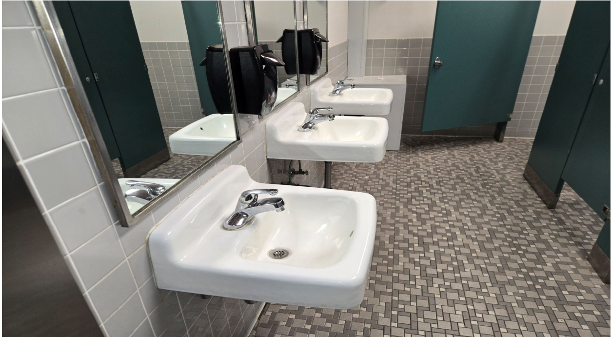
Photograph 1 - Typical Lead-Coating on Sinks Located Throughout Restrooms of Building.
